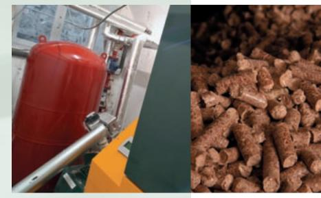
The output of the boiler can be adjusted to the heating requirements, in a fully automatic way, from stand-by to full-load operation. The pellet boiler is connected to the 5000 litre hot water storage tank (see heating and cooling section on pages 8-9) and the boiler heats the main building of the Renewable Energy House.
